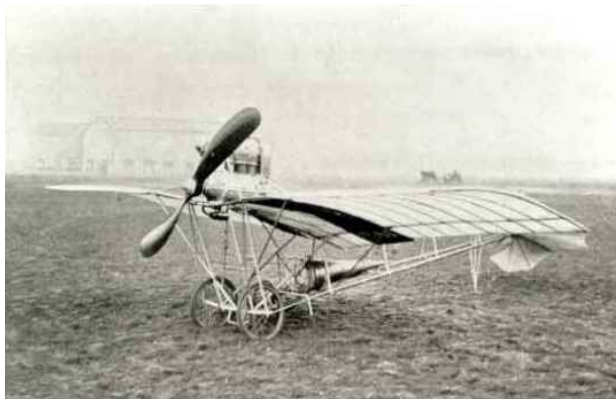
Figure 2.1: Santos Dumont's Demoiselle. Generally considered the first minimum aeroplane. Fuselage constructed from bamboo (presumably in lieu of decent aluminium alloy tube!).
